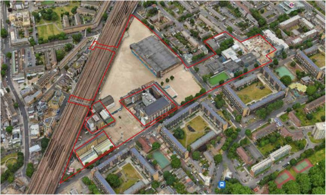
Aerial photo taken in 2022 showing the cleared parts of the site at that time, the new school under construction, the Workspace buildings outside the application site and the surrounding area
